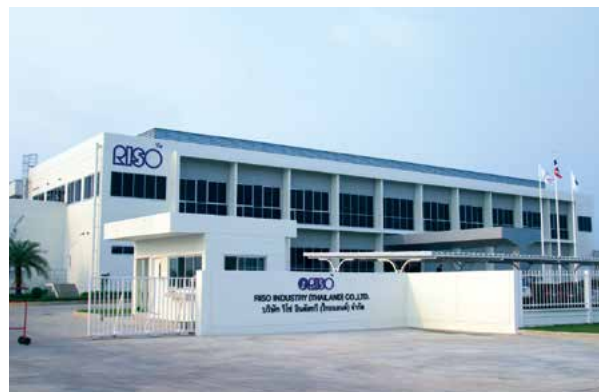
RISO INDUSTRY (THAILAND) CO., LTD. new plant (Ayutthaya, Thailand)
