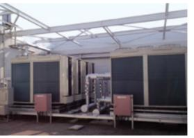
Introduction of highly efficient hot/cold water heat pump chiller (Ube Plant
